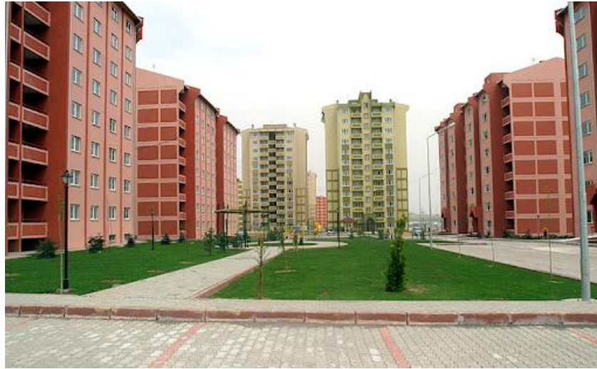
b) Halkalı Housing Project
